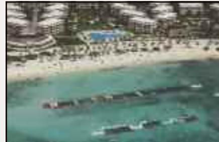
Geotube® unit placed offshore for use as a breakwater.
