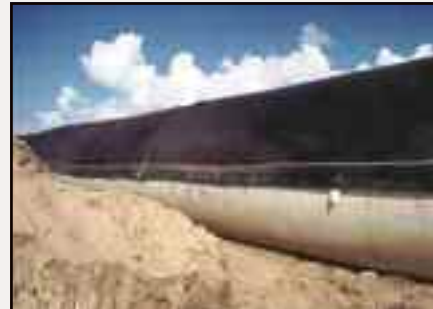
Protective cover shields Geotube® containers from sun's damaging UV rays.
