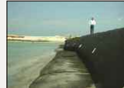
Geotube® containers are stacked to produce this protective structure.
