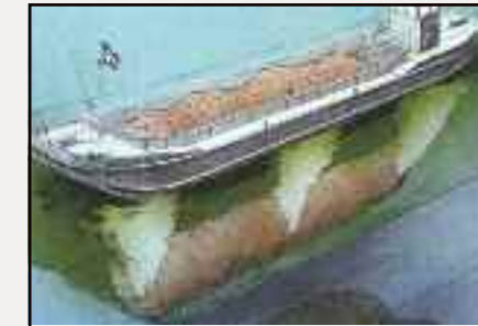
Geocontainer® unit being dropped from split bottomed barge.
