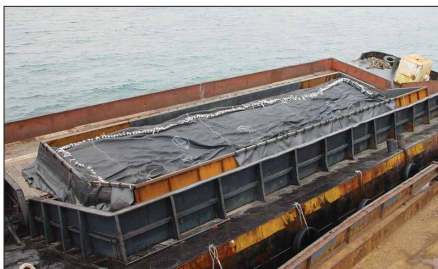
Geocontainer® offshore breakwater construction
