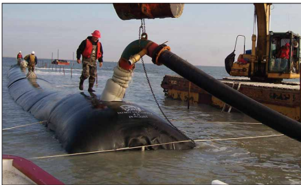
Geotube® containment dyke construction
