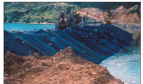
Mirafi® FM geotextile behind rock containment dyke
