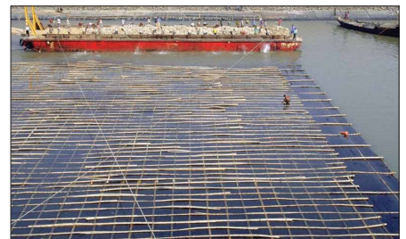
Mirafi® FM geotextile beneath rock bed protection
