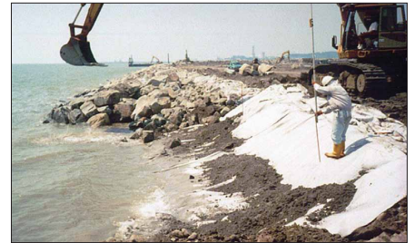
Polyfelt® F filtration geotextile beneath rock revetment
