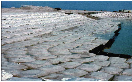
Geobag® revetment construction
