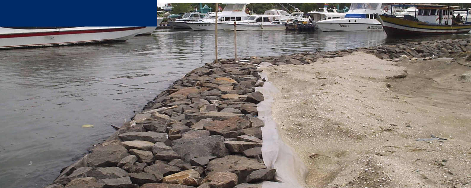
Rubble containment dyke with geotextile filter
